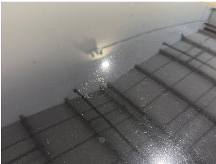
15: Roof Scratched Over 25mm Thru Paint
