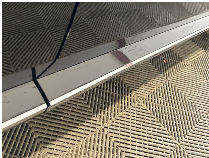
2: Door osf Chipped Edge Chip
