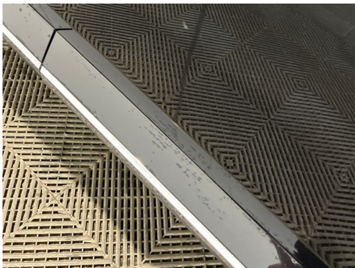
1: Door osf Chipped 1 To 5
