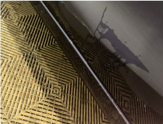
11: Door nsr Dented With Paint Damage
