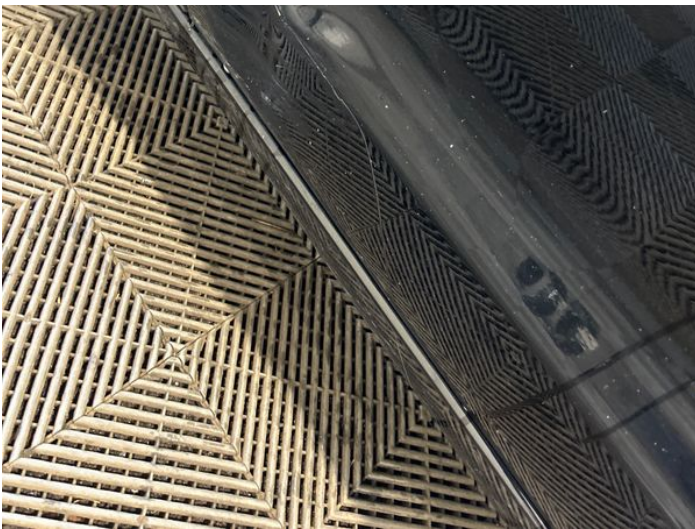
11: Door nsf Dented With Paint Damage
