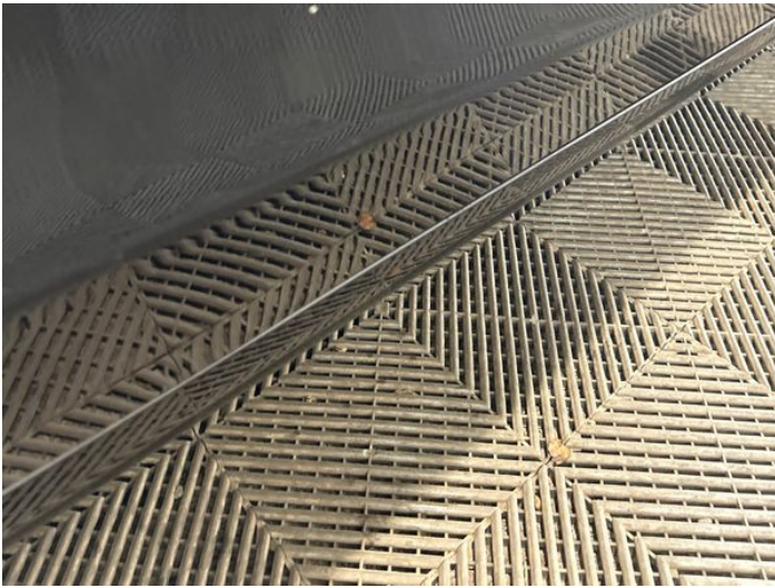
5: Door osf Chipped 1 To 5
