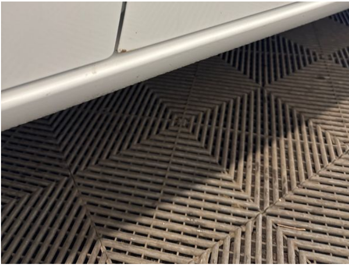
17: Door osf Rusted Over 5mm
