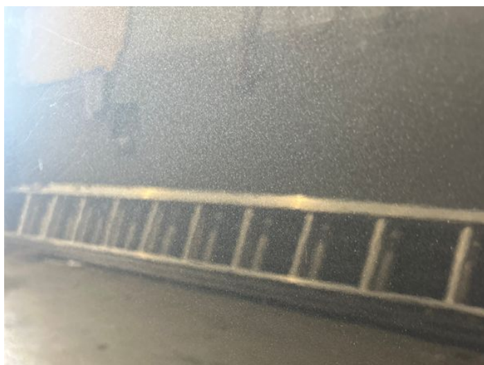
8: Door nsr Chipped 1 To 5
