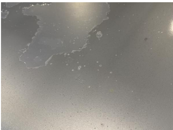
7: Roof Poor Previous Repair Paint Flake
