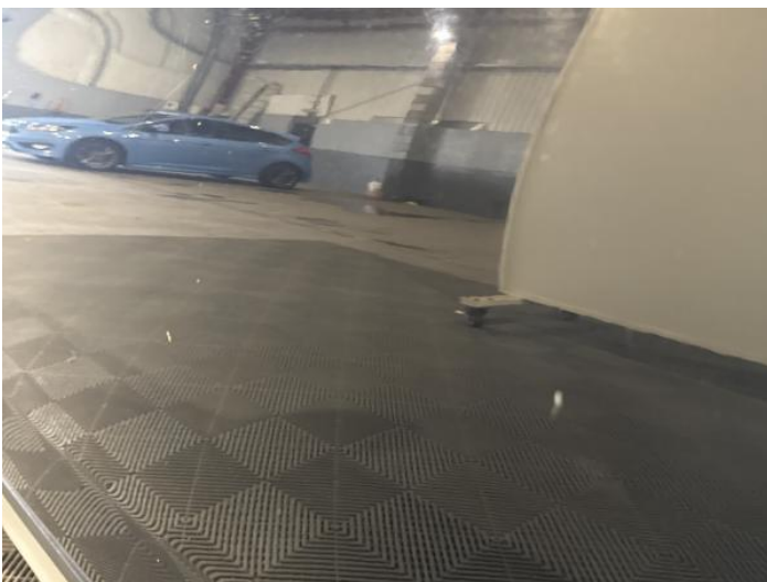
7: Door nsf Chipped Multiple Chips
