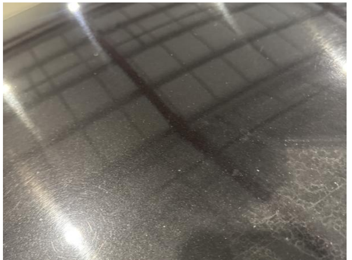
18: Roof Dented Between 10mm + 30mm
