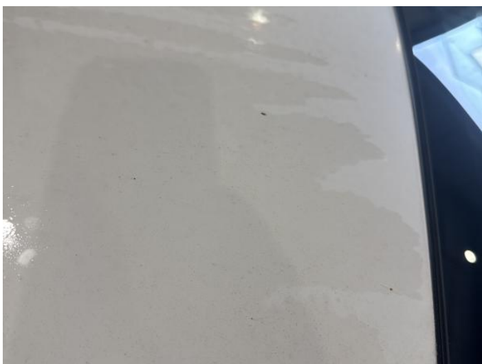
13: Roof Chipped 1 To 5
