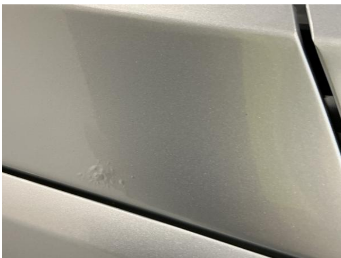
25: A Post os Rusted UpTo 5mm
