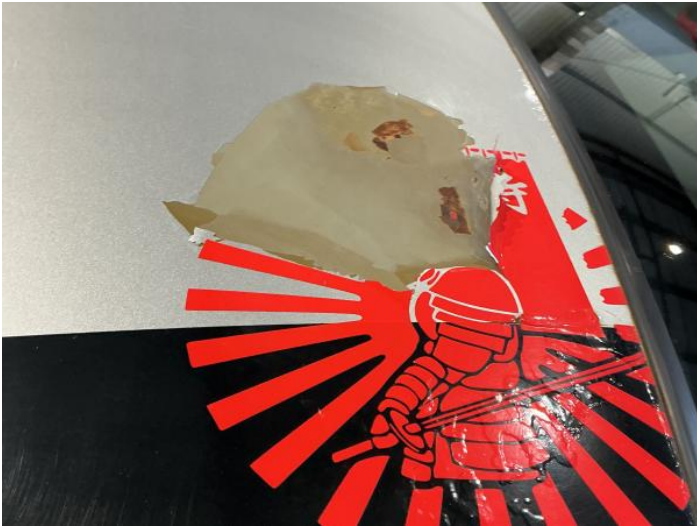
15: Roof Poor Previous Repair Paint Flake
