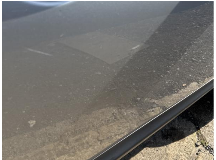
6: Door osf Scratched Over 25mm Thru Paint
