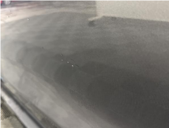
3: Door nsf Chipped 1 To 5
