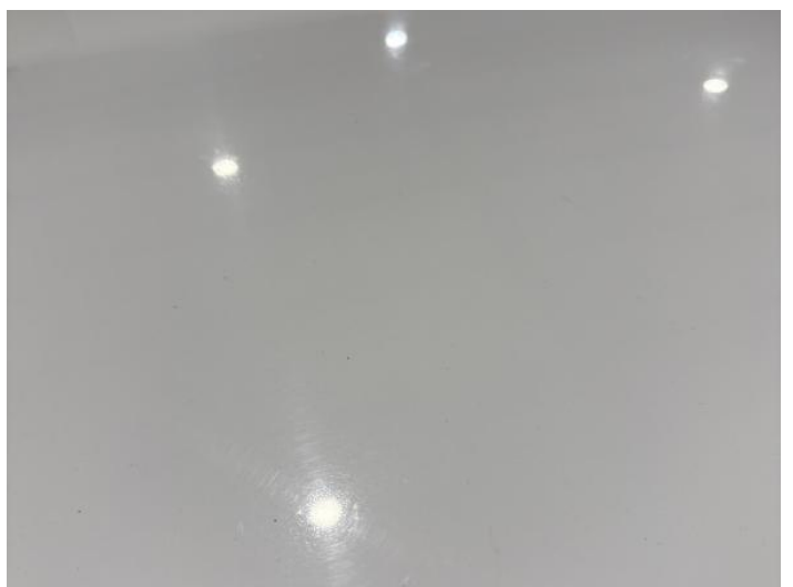
14: Roof Dented 2 Or Less UpTo 10mm
