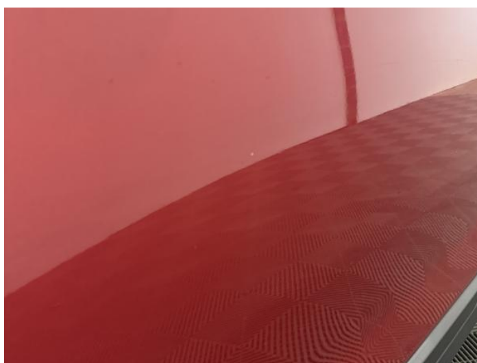
14: Door osr Chipped 1 To 5
