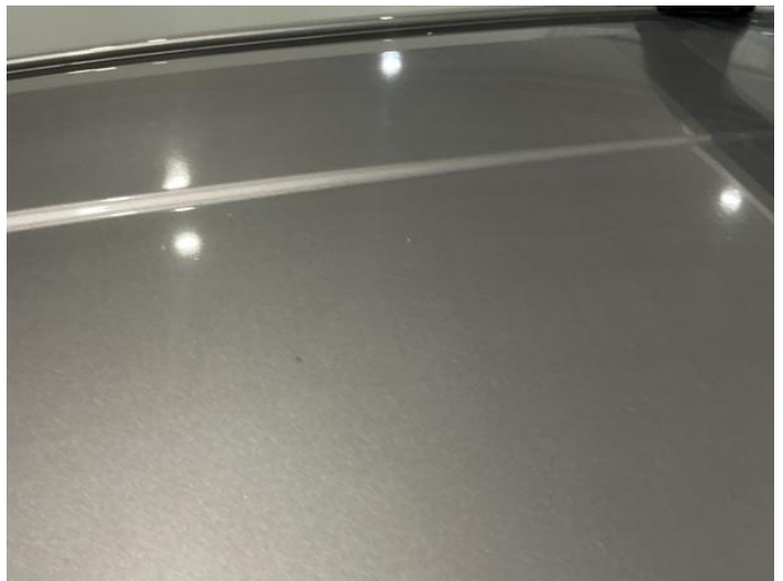
12: Roof Dented Between 10mm + 30mm
