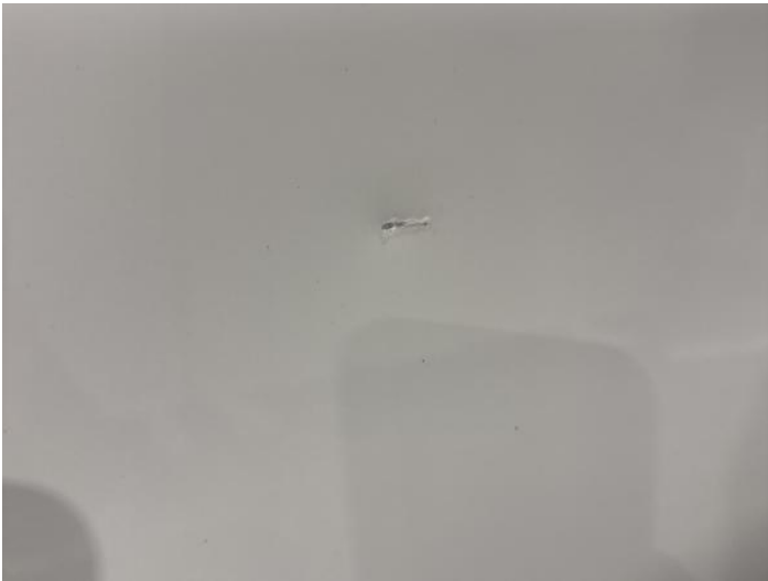
5: Door nsr Scratched UpTo 25mm Thru Paint
