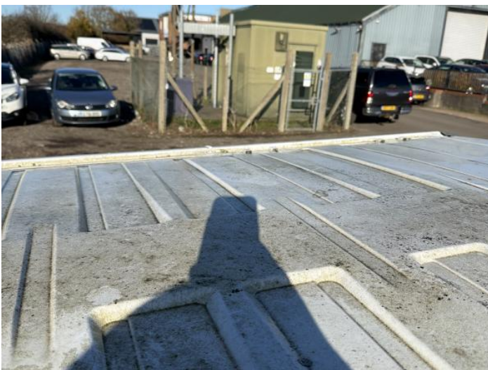
13: Roof Dented Over 30mm
