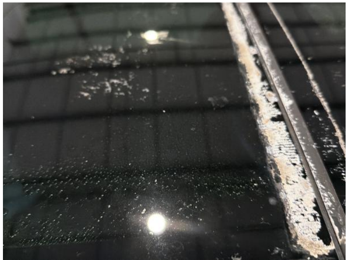
18: Roof Poor Previous Repair Poor Paint
