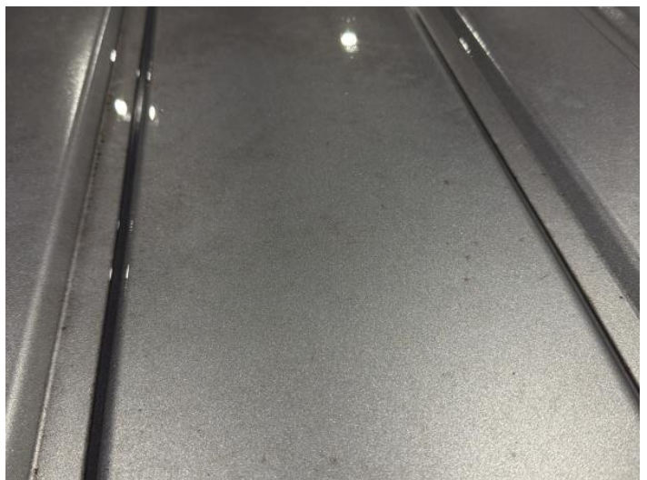
20: Roof Dented Over 30mm
