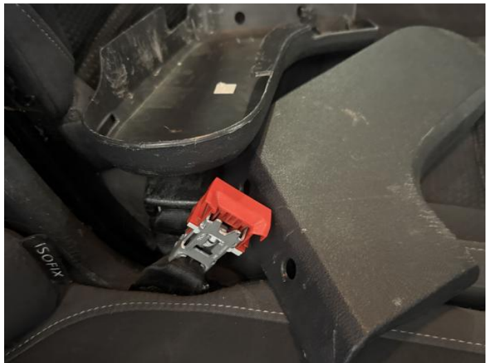
2: Seat Belt osr Broken Replace
