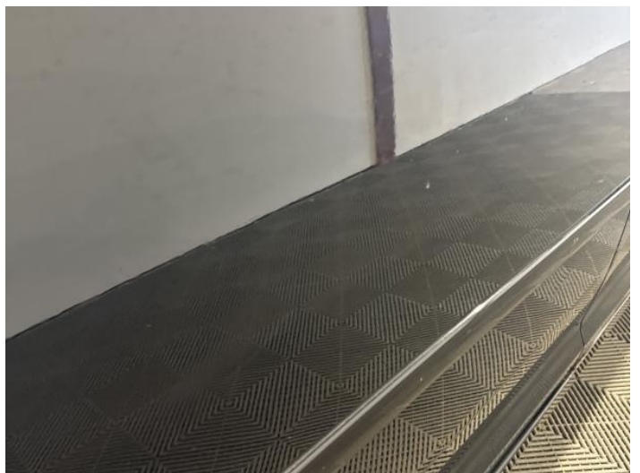
20: Door osr Scratched Over 25mm Thru Paint
