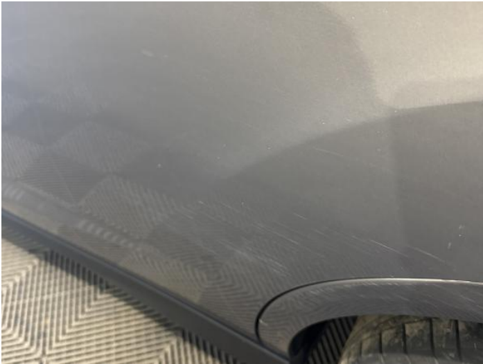
9: Door nsr Scratched Over 25mm Thru Paint
