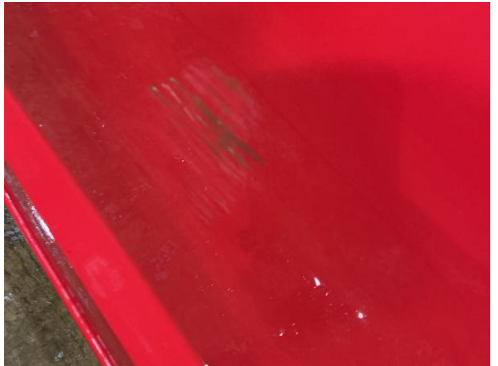
2: Door osf Scratched Over 25mm Thru Paint
