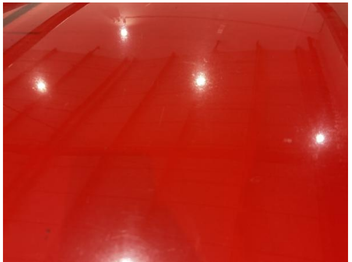
18: Roof Scratched Over 25mm Not Thru Paint
