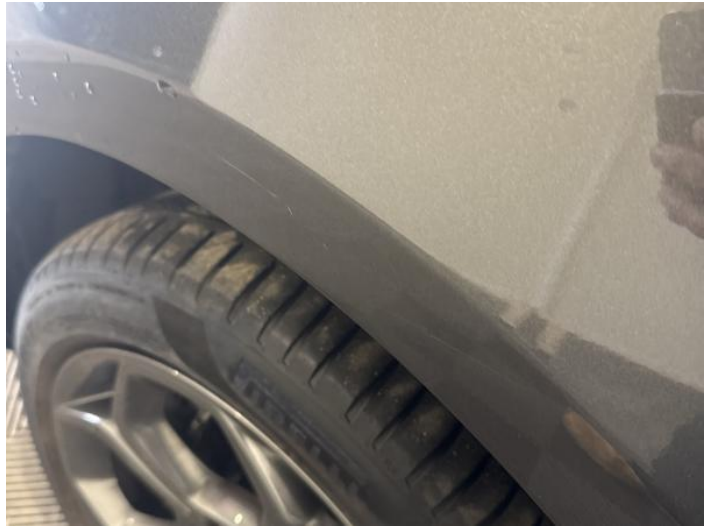
4: Wing nsf Scratched Over 25mm Thru Paint
