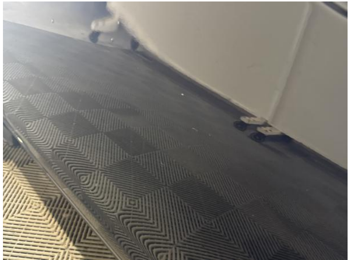
6: Door nsf Chipped Multiple Chips
