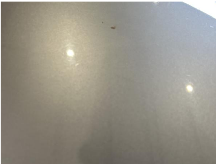
17: Roof Chipped 1 To 5
