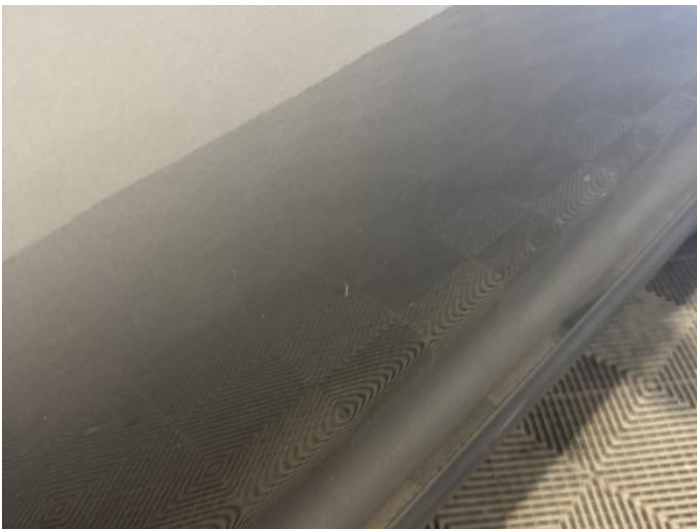
11: Door osf Chipped 1 To 5
