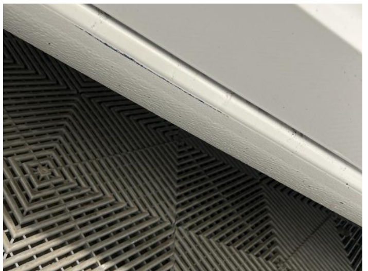
14: Sill os Scratched Over 25mm Not Thru Paint
