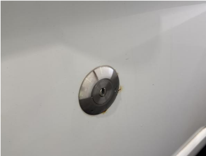
15: Door osf Rusted Over 5mm
